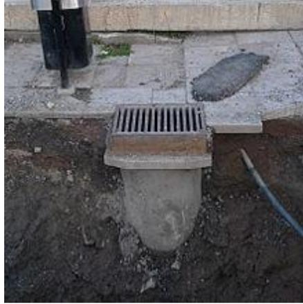
Storm drain with pipes visible beneath it during construction work
