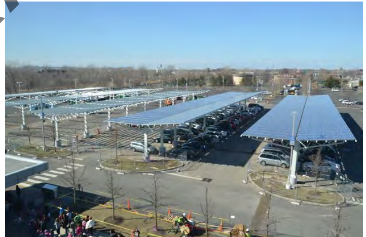
Figure 51. Solar canopies over parking at the Liberty Science Center. Source: LSC.org, "LSC is going green(er)".
